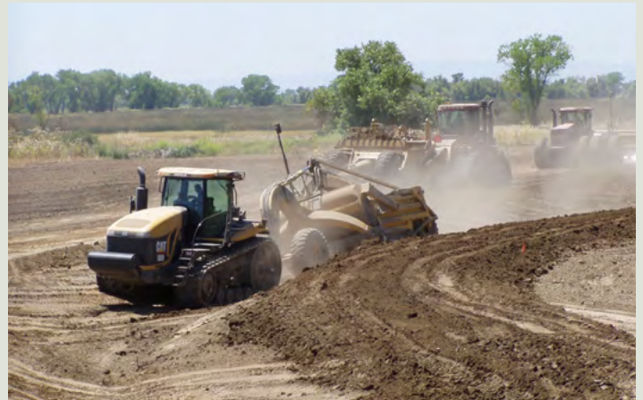
Levee construction for wetland habitat restoration, Gray Lodge Wildlife Area - Ducks Unlimited, Inc.
