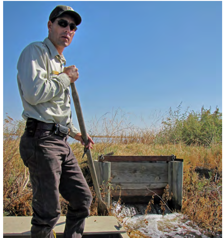
Manager checking a water control structure at Twin Lakes Partners for Fish and Wildlife project - Shawn Milar
